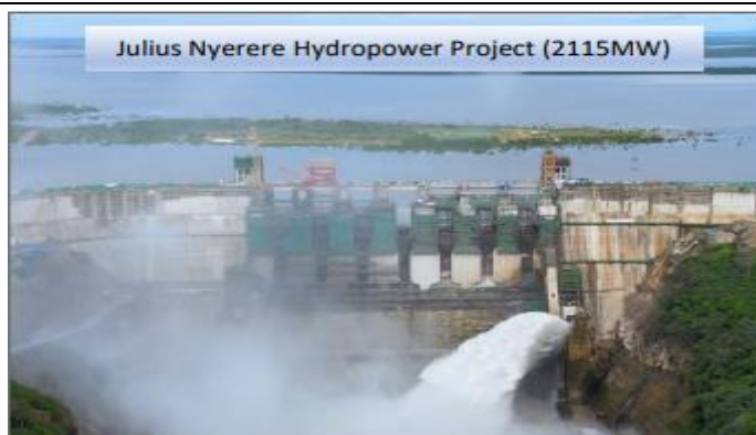
Figure 18: Julius Nyerere Hydropower Project (2115MW)
