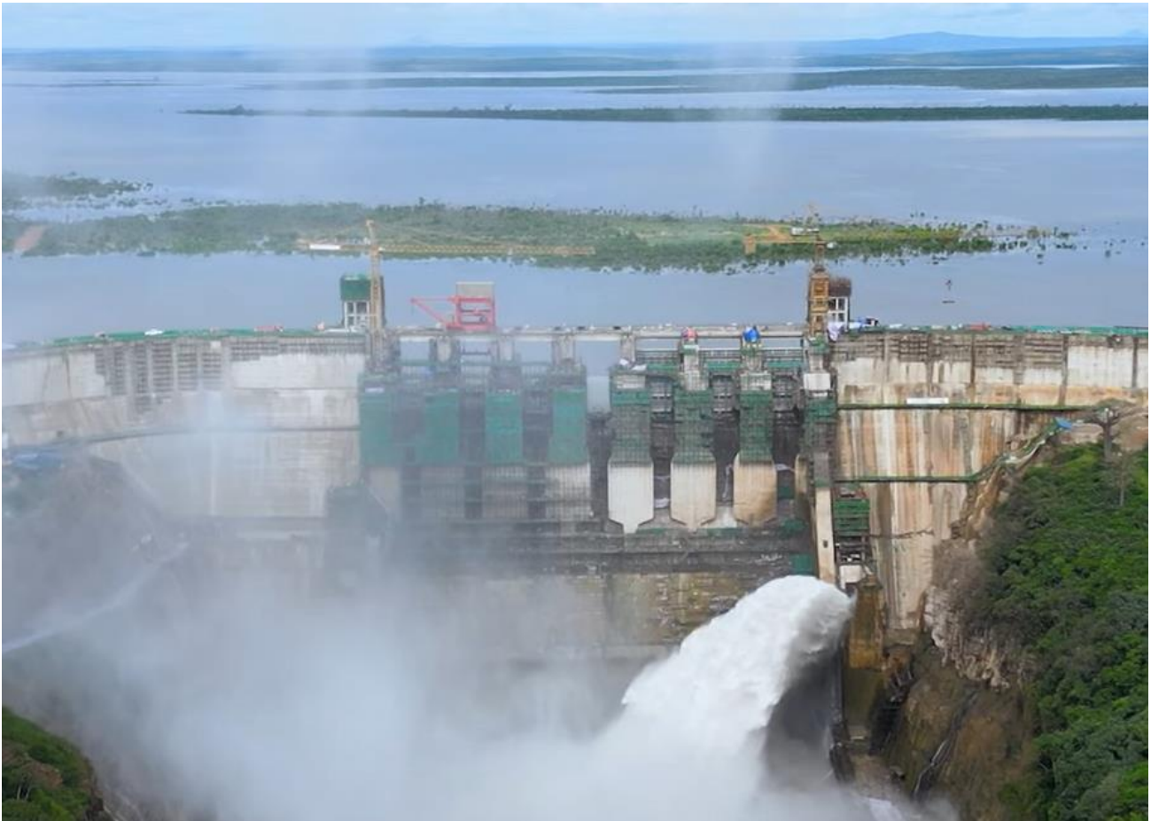
Photo 1 - The 2115MW Julius Nyerere Hydropower Project is expected to begin power generation soon
