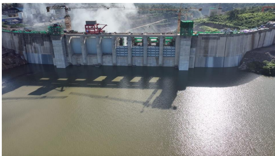
Figure 2: Julius Nyerere Hydropower Station planned for commissioning in mid-2024
